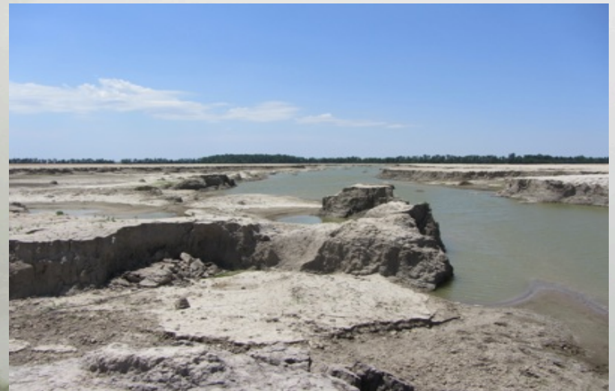
Photos of BPNM Floodway scouring and deposition, 15 th June 2011
